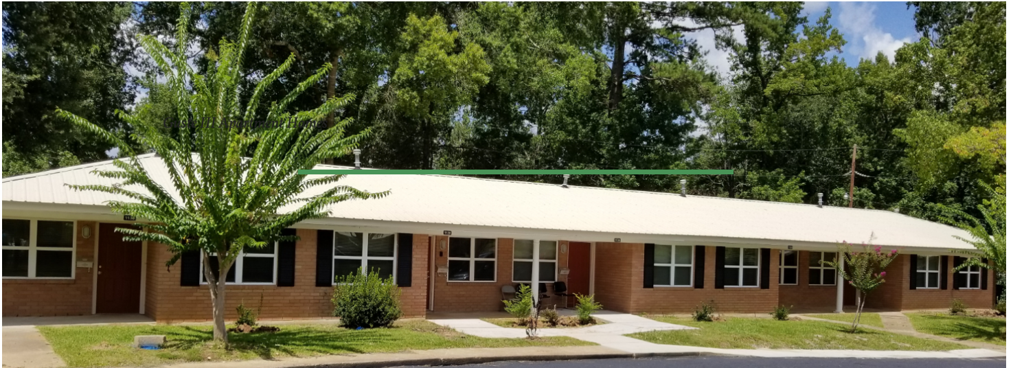
Newly Renovated Logan Lane Site at Twin Lakes of Leesville
